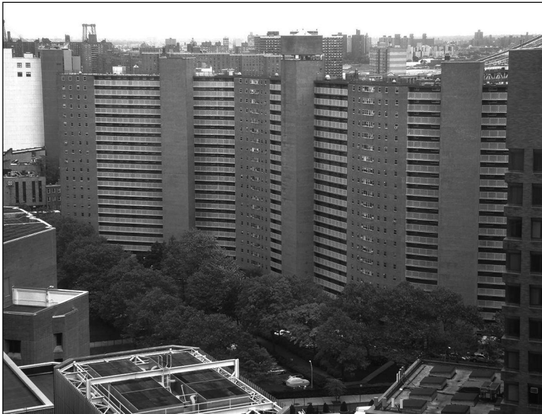
Articulated elevator towers leading to open corridors on the west facade of Chatham Green provide vertical overlay to the stacked apartment floors.
