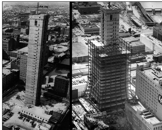
Lincoln First Tower: John Graham Company's tower design started with a concrete core but switched to steel to form the external structure with its signature flaring base.
