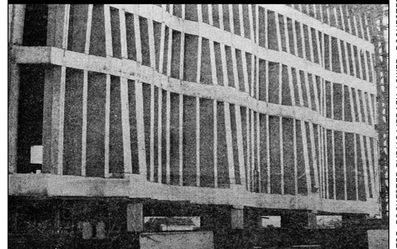
Marine Midland: The lower image shows Khan's solution of variable column thickness to achieve the load transfer at the base.
