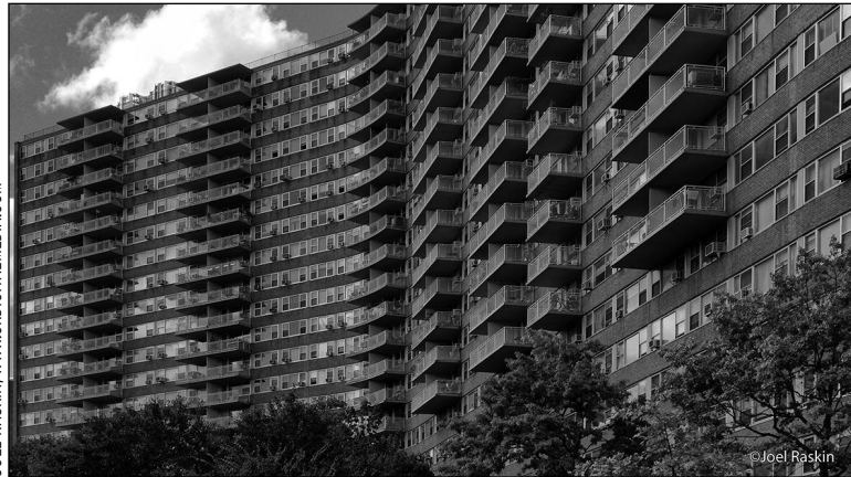
Ribbons of windows and balconies alternate with those of brick on the east facade.
